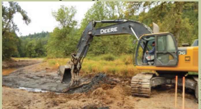
Installation of an engineered log jam.
