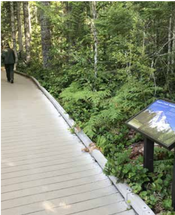
Boardwalks and well-placed interpretive panels, such as those shown here in Mount Rainier National Park, can reduce impacts on sensitive resources while enhancing the overall visitor experience. Credit: National Park Service, Digital Assets Management System
