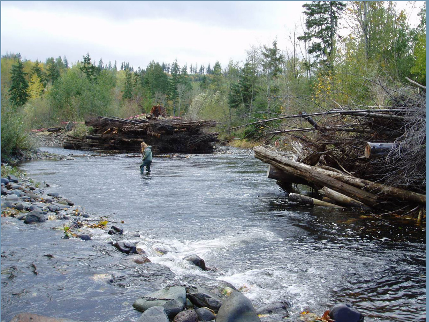
Engineered logjams, pioneered by the Tribe's Department of Natural Resources to improve salmon habitat on the Mashel River (above), are now used throughout the Pacific Northwest.
