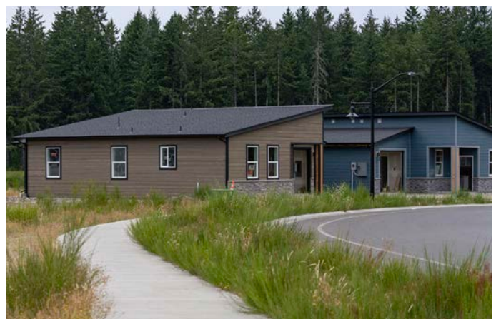
The Tribe will install solar panels and backup batteries on its new Elders Village homes. The Tribe should also incorporate clean-energy systems and energy efficiency into the retrofitting of existing residential buildings.
