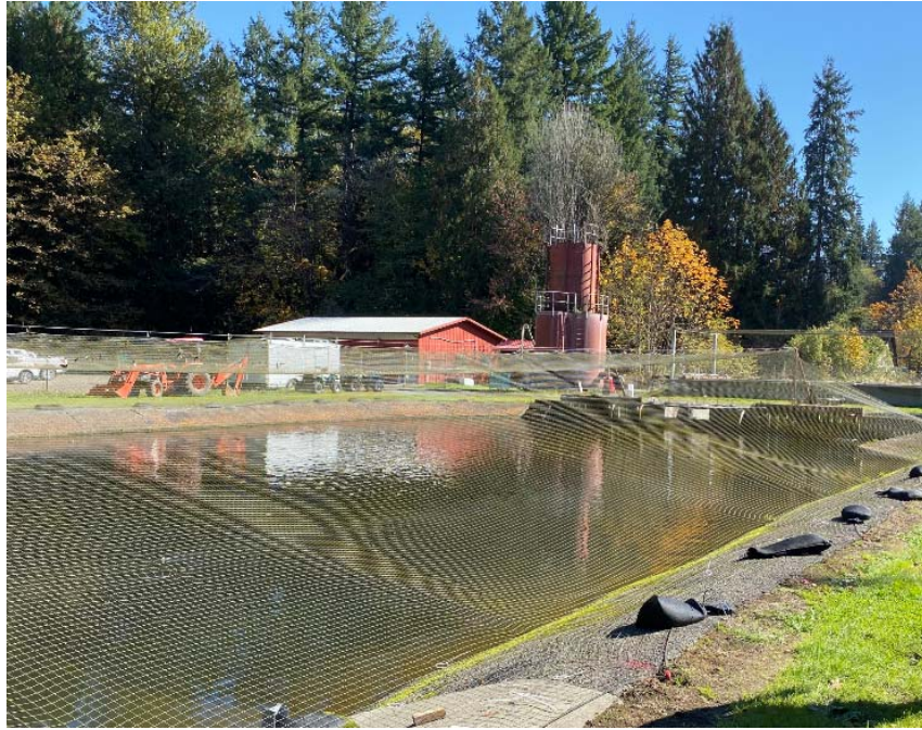
Plate 1. Upper site with holding pond, headtank, office building, and concrete raceways in view, looking east.
