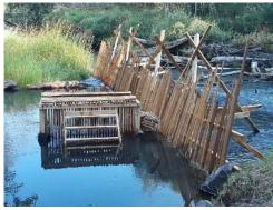
position in the main stem would require constant maintenance due to the force of main stem flow. The weir was determined that it could be used in a hatchery creek to harvest excess hatchery rack.
